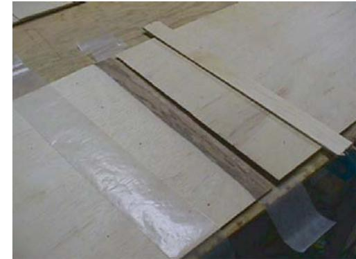
Some individuals prefer to use a butt joint. Quicker and easier but not as pretty. It is also more difficult to hide. To use a butt joint, simply butt the two ends together and fiber glass both sides with cloth four to five inches wide.
